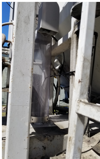
Extending the discharge chute with 5 in clear tubing.
