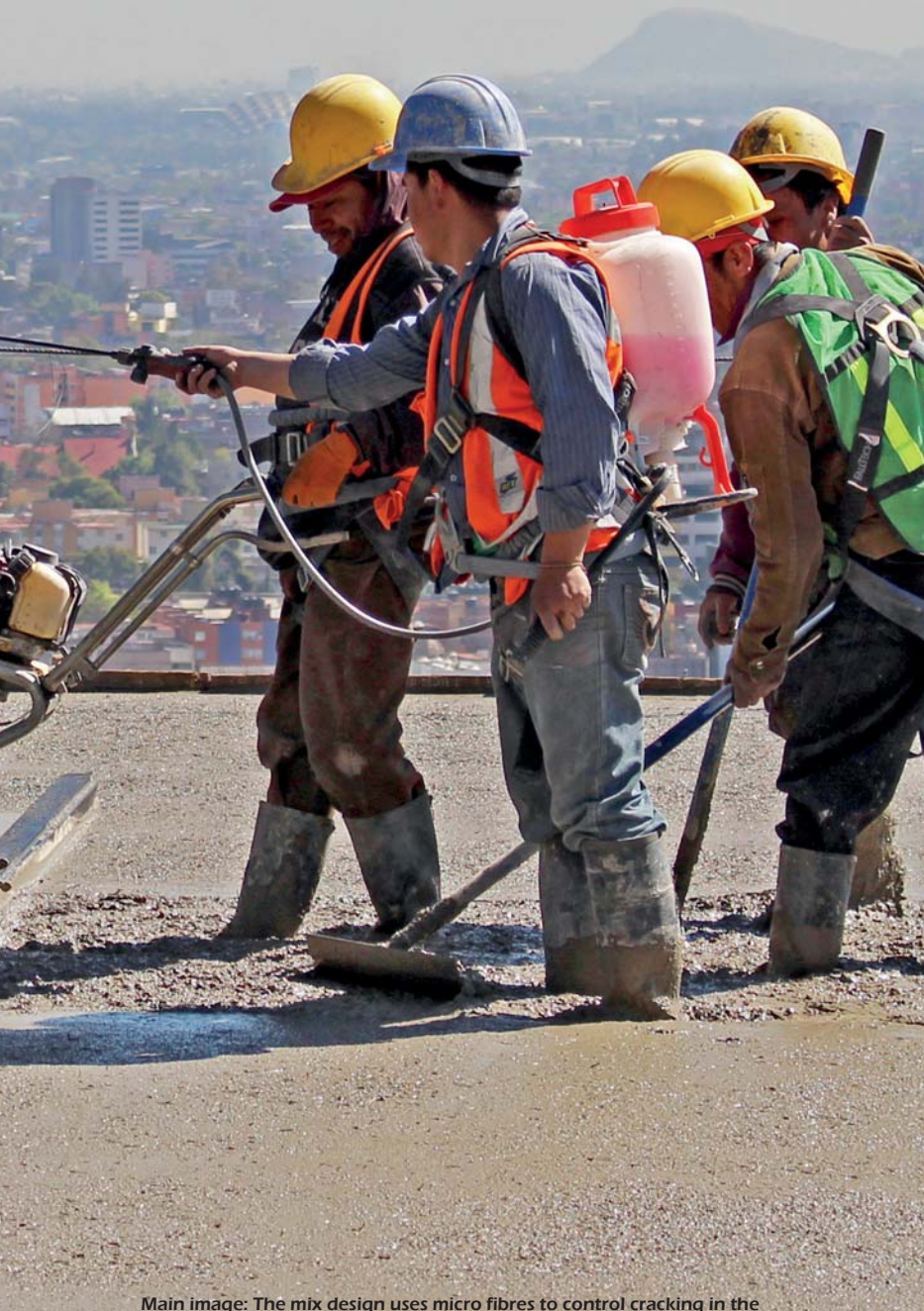
Main image: The mix design uses micro fibres to control cracking in the slabs. Inset, right: The finished tower will cover 5600m 2 of floor space. Below: A ProAll Reimer Mixer is loaded with stone and sand while pouring at the base of the building.
