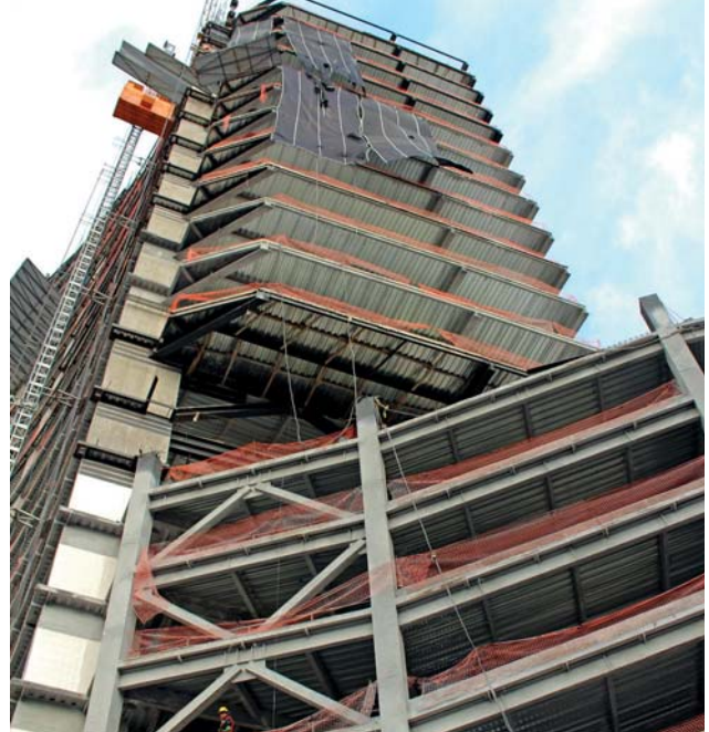
Above: The 25-storey building has been under construction since 2014.
